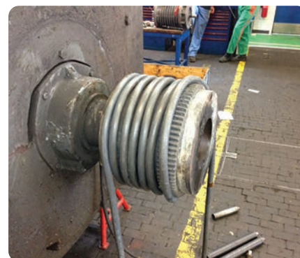
Heating a coupling for dismounting
